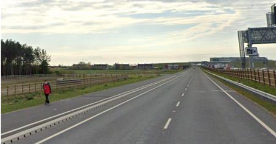
Local Access road NMU facility
